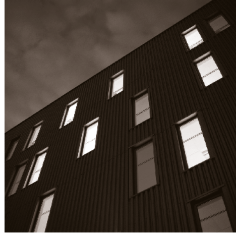
Figure 5. Exterior detail at night: The façade of the administrative building, which faces a busy and noisy motorway, displays a jewel-like presence at night.
